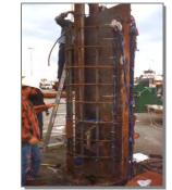
An O-cell assembly is prepared for installation using two 4 MN (900 kip) cells for use in a 1200 mm (48") diameter shaft.
