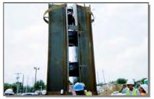
Two 16 MN (3600 kip) O-cells used to test the lateral stiffness of the Cooper Marl (between19-21 m depth) on a 2400 mm (96") pile for the Cooper River Bridge
